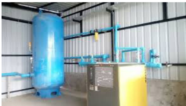
Figure 47: HDPE Aluminium Pipe-line
